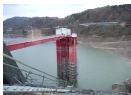
Selective water intake system
