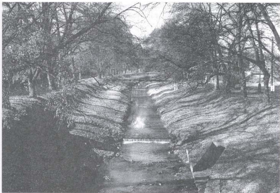
Photo 1 Section (no. 6) river training of the Rakovnický Stream
