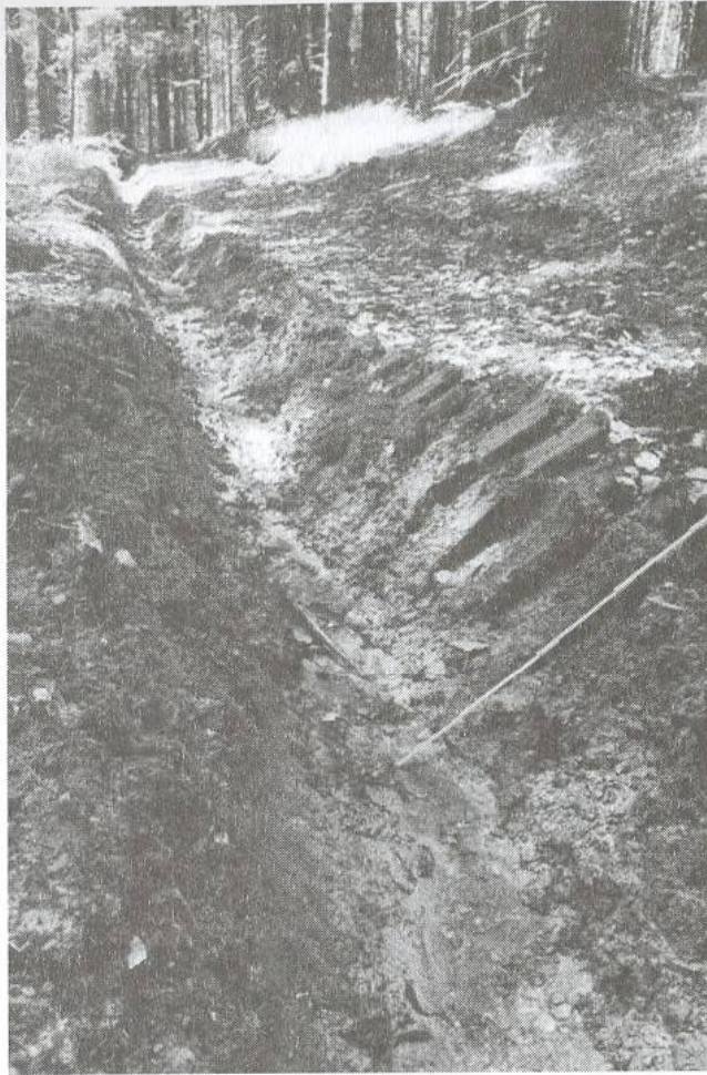
Photo 1 Furrow caused by tractor wheels on the forest road surface, deepened by linear drainage
