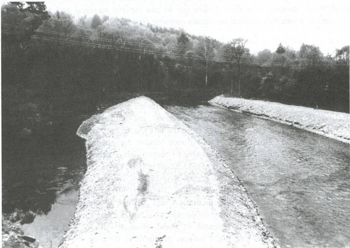
Photo 3. An example of wrong localised levees by Nové Heřminovy (Photo V. Vilímek)
