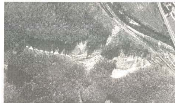
► Photo 6 Active slope deformations in the Bystřička area
