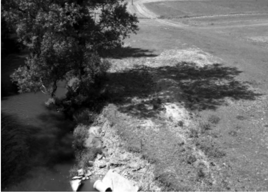
Fig. 8: The bank scour and flood overbank accumulation behind a bridge below Havlíčkův Brod. The bridge and its road create a transverse barrier in Sázava River floodplain
