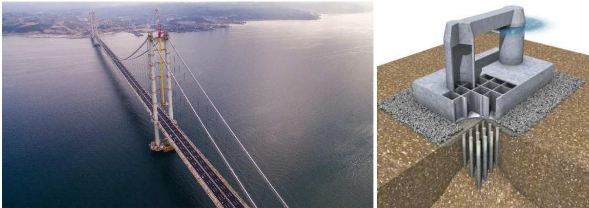
Figure 6. (a) Aerial view of completed bridge; (b) Foundation principle for tower foundations with inclusion piles
