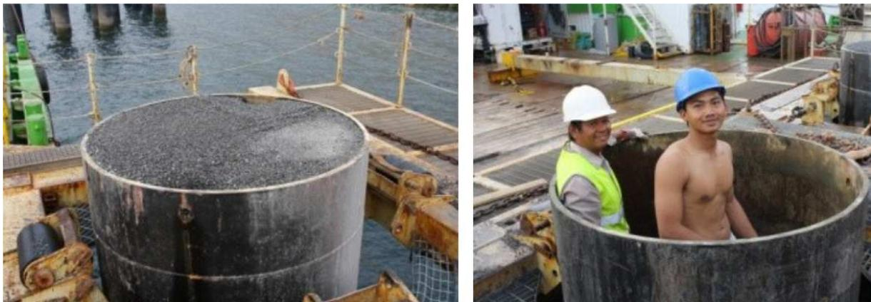
Figure 4. (a) Pile with gravel surface after final driving, (b) gravel excavation and preparation for casting of concrete on top of gravel
