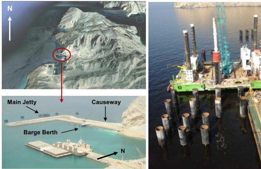
Figure 3. (a) Location and overall layout of facility; (b) Driving of piles in progress
