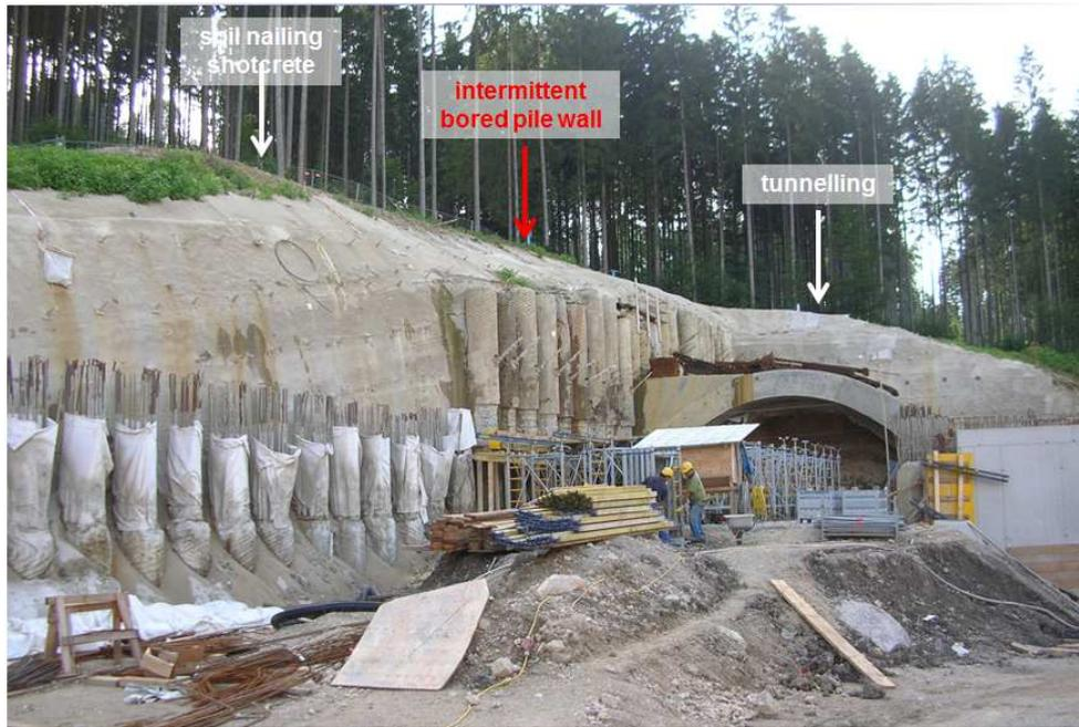
Fig. 6. City Tunnel Waidhofen an der Ybbs. Construction phase. Open cut and cut-and-cover section in creeping slope. Retaining structure made of intermittent bored pile wall (diameter 90 cm, axial spacing 1.39 m, pile length about 20 m) anchored with pre-stressed anchors (Photo: Dietmar Adam/Roman Markiewicz).
