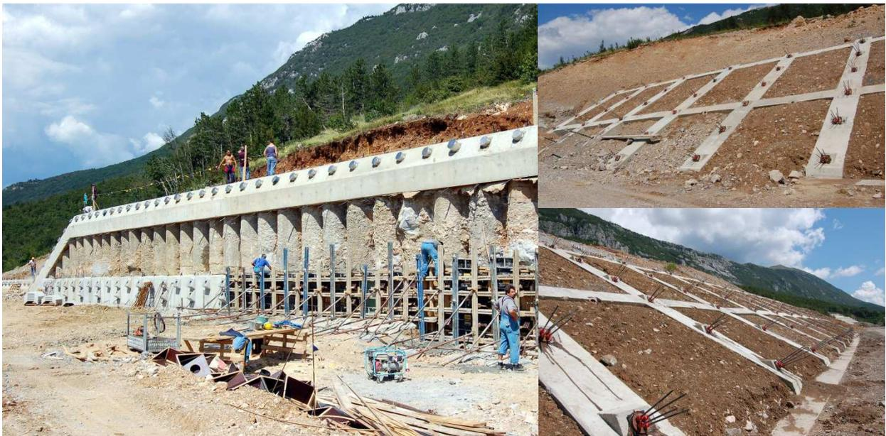
Fig. 9. Rebernice Landslide. Construction phase. Anchored bored pile wall linked by cap beam (left) and pre-stressed anchored reinforced concrete grid beam structure (right) (Photos: Boštjan Pulko).
