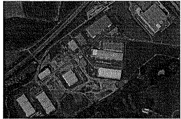
Abb. 4: Logistikpark Rudná (Geodis Brno)
