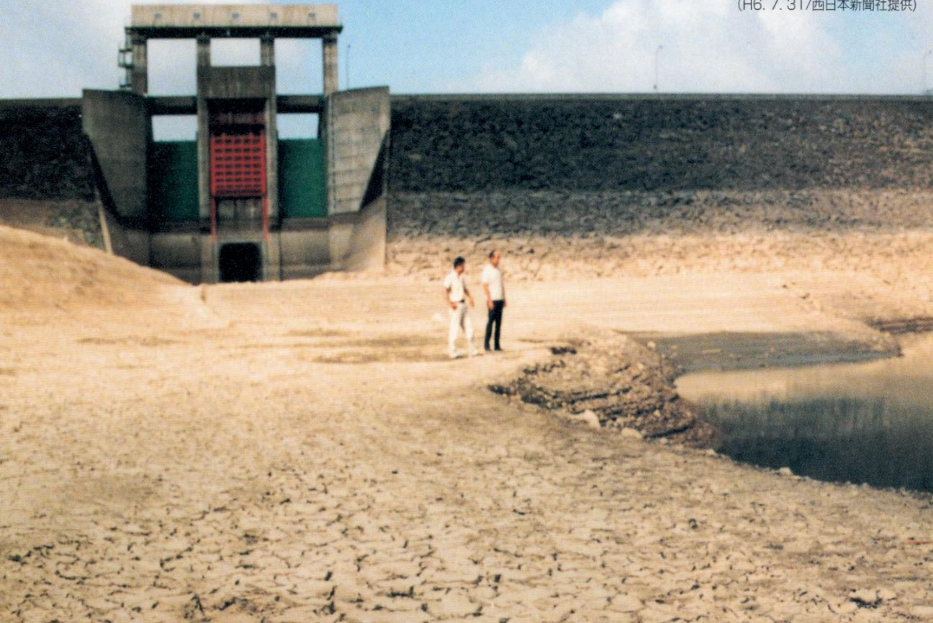
Drying up SAMEURA Dam in Kochi, Japan (31 July 1994)
