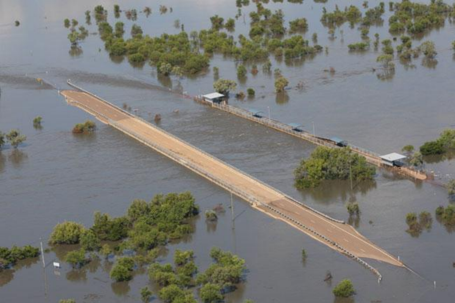
Normanton to Karumba Road cut, February 2010
