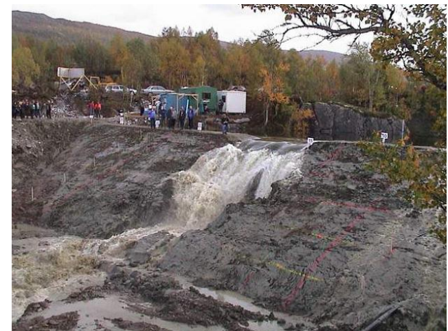
Photos from FLOODsite
