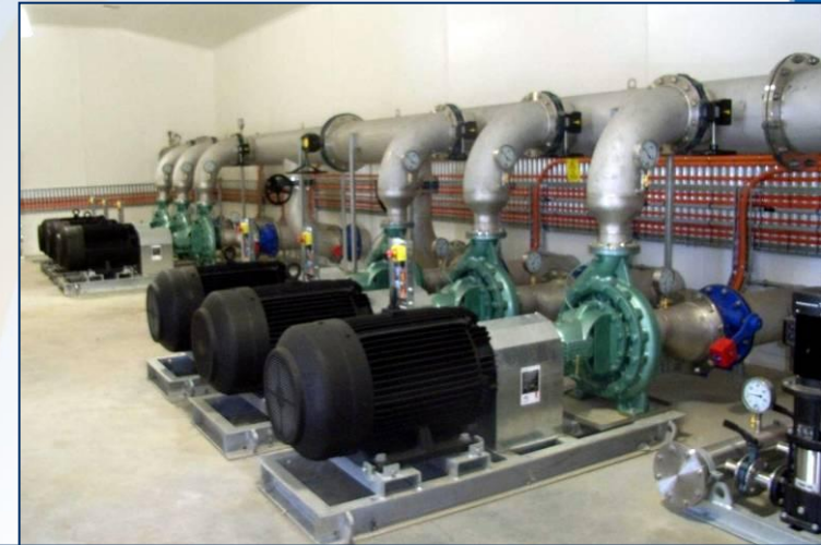
Typical Pump Station
