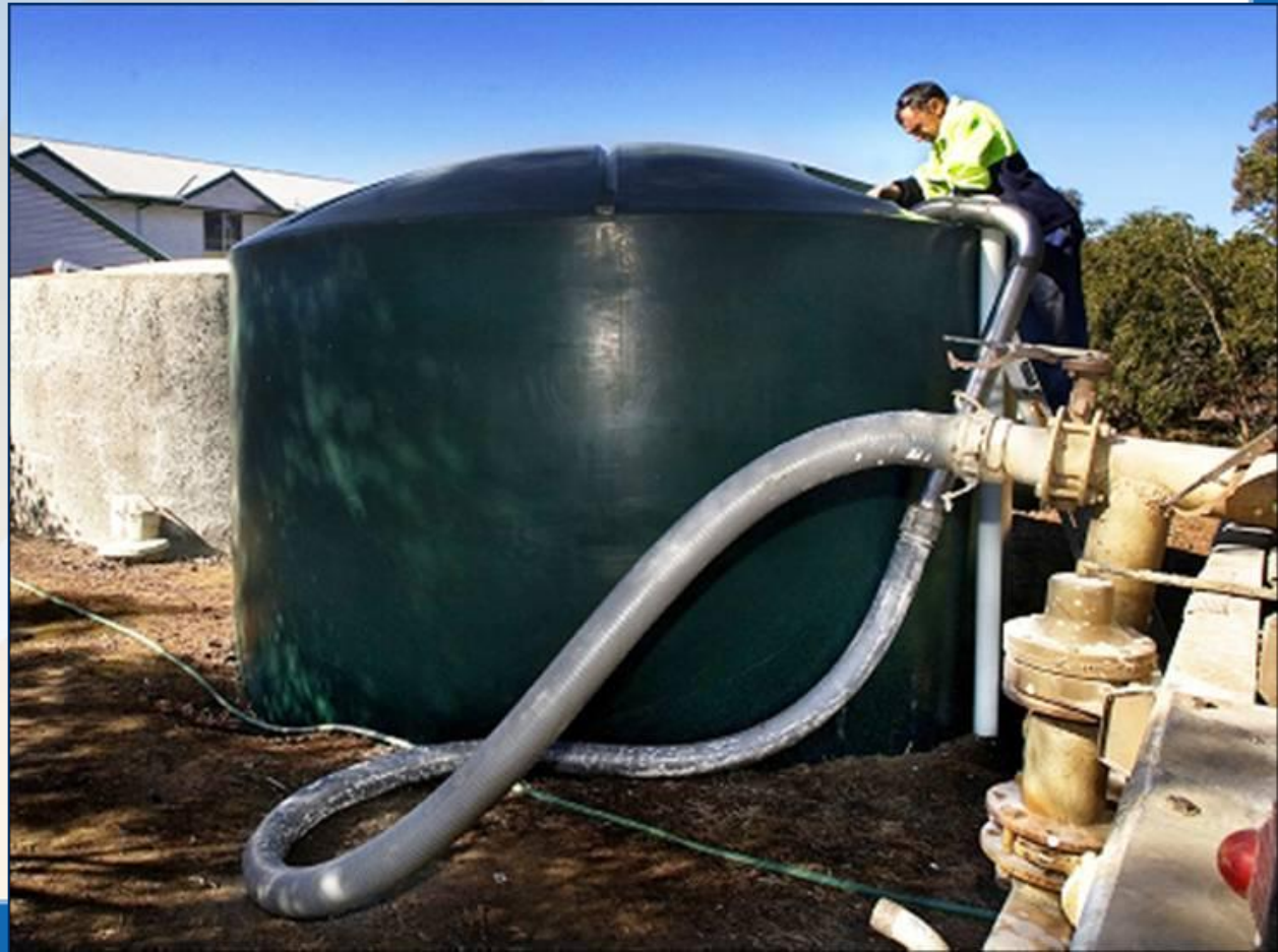
Domestic Tank Being Filled
