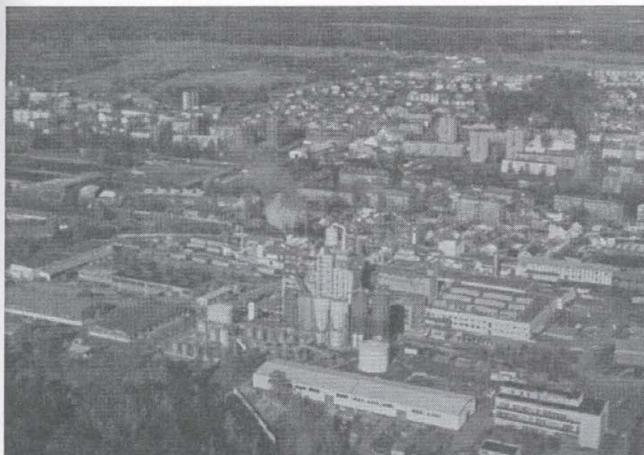
Photo 3 Rakovník – Procter & Gamble chemical plant
