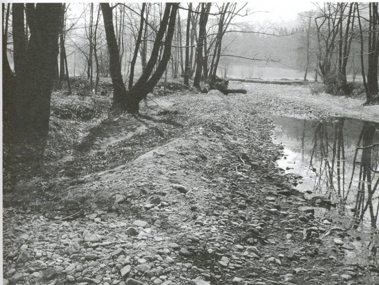
Photo 1 Abandoned river bed of the Volyňka river (near Malenice). Shifted river bed of the Volyňka river was formed in consequence of the cracking of its right bank, which was weakened by mining of river sands (Photo by Z. Engel, 2003)
