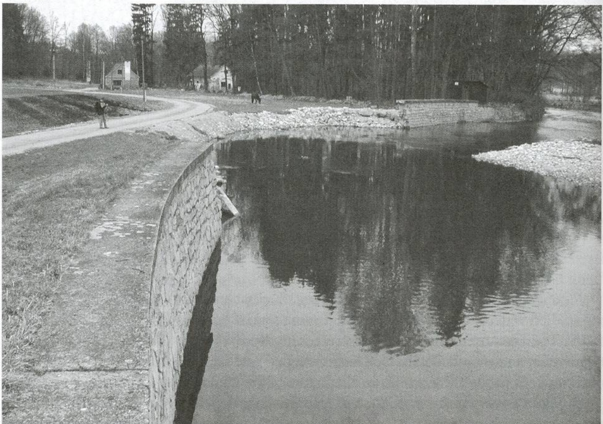
Photo 2 Broken flood-control levee in the Volyňka river near Volyně. During the flooding the main stream headed straight to houses (Photo by Z. Engel, 2003)
