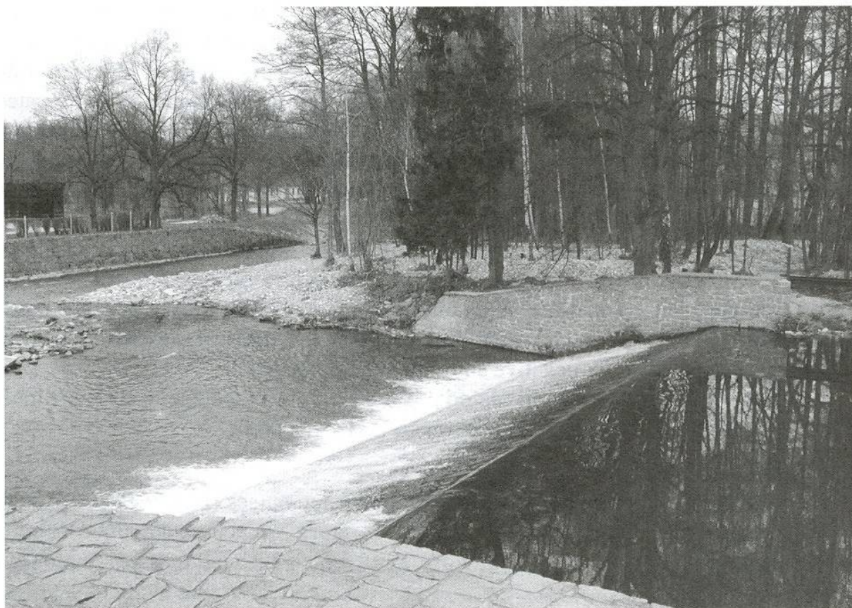
Photo 3 Surroundings of weirs are dangerous and more prone to overspill due to water flow. This location of weir near Volyně is good example of total ignorance of natural principle of water circulation in case high flow rate of water. This weir is situated in front of orthogonal bight of river. Gravel-stony accumulations on the bank are a proof of the lapse of the purpose of this weir and the threat of neighbourhood localities by deflected main stream of the Volyňka river (Photo by M. Křížek, 2003)
