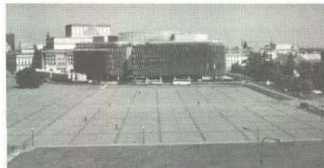
Fig. 5 The Metropolitan office building (construction in 2001–2003, design by Sir N. Foster)
