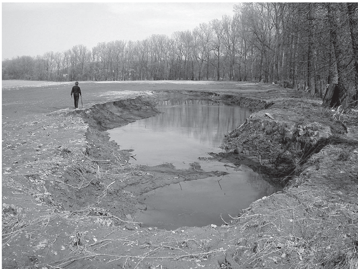
Fig. 5 Intensive erosion in floodplain in central Sázava course by Poříčí nad Sázavou. The improper use of the floodplain helps to accelerate the geomorphological processes during the flood and leads to rise of the direct as well as secondary flood damages. Photo V. Vilímek, 2006
