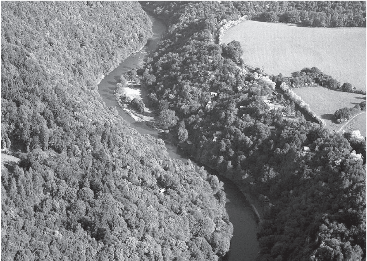
Fig. 1 Deep valley of Sázava River on the down course does not allow important anthropogenic transformation in terms of stream route or riverbed modification. However the weirs and natural steps in the riverbed occur frequently in this part of the river. Photo M. Raudenský, 2006
