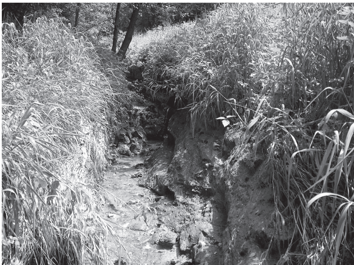
Photo 2 Intensive erosion at the margin of the floodplain (up to the depth of 1 m).
