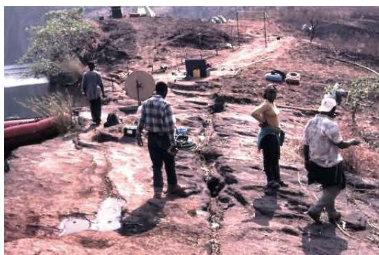
Fig. 5. Fractures in the pyroclastic dam at Lake Nyos.
