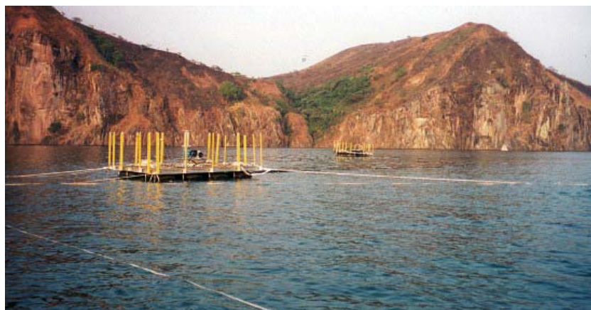
Fig. 7. Raft supporting the pipe at Nyos. Control equipment on raft in the background.
