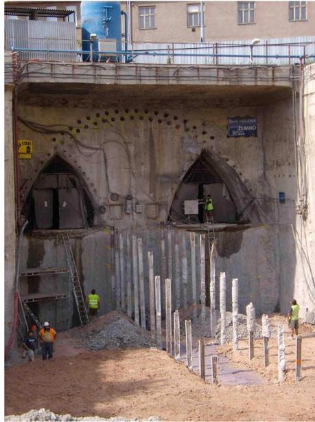
Figure 4.6: Exploratory adits situated in the top heading of the future Dobrovského tunnel.
