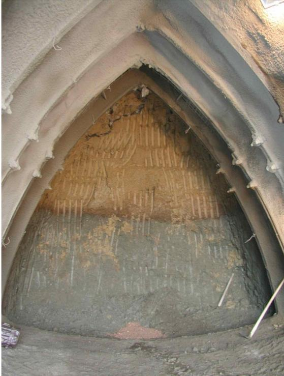
Figure 1. Exploratory adit of Dobrovského tunnels showing transition of weathered and sound Brno clay (Pavlík et al., 2004).
