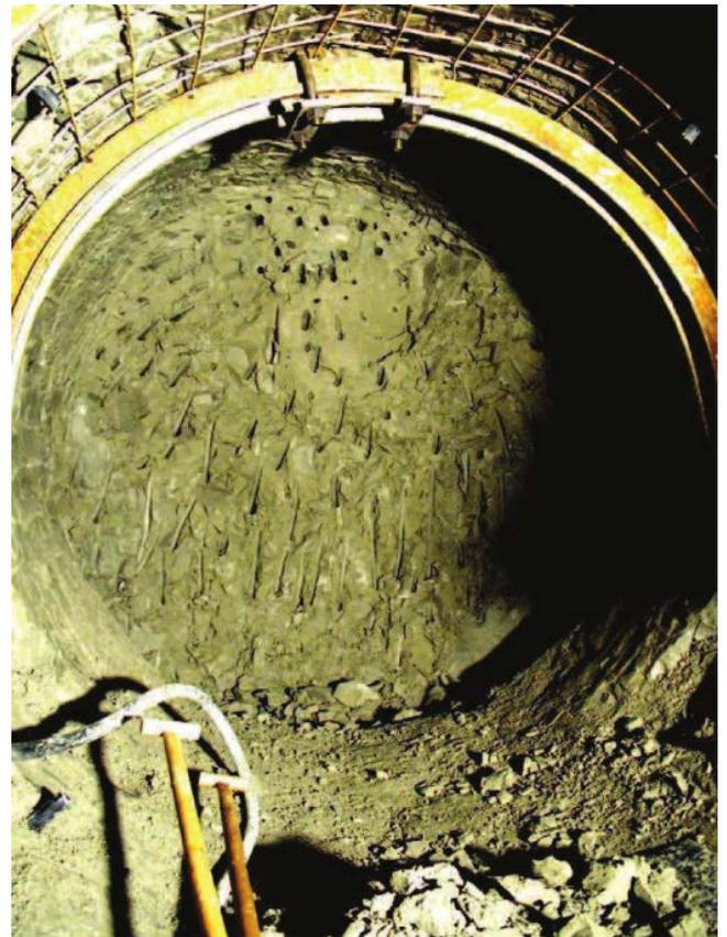
Figure 4. Safety support of the circular adit R2 (Pavlík et al., 2004).
