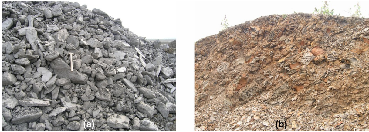
Fig. 2: Landfill during construction (a) and after 15 years of self-weight consolidation and weathering (b).
