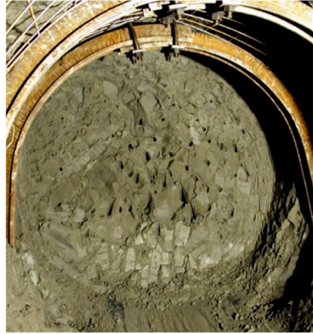
Figure 4a and 4b. View at the excavation face of exploratory gallery IIB (Figure 4a) and unsupported adit R2 (Figure 4b), Pavlík et al. 2004.
