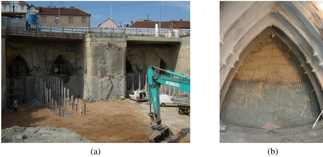
Figure 3: (a) Exploratory drifts situated in the top headings of the future Královo Pole tunnels; (b) detail of the drift with the boundary between weathered and non-weathered Brno clay (Pavlík et al. [28]).
