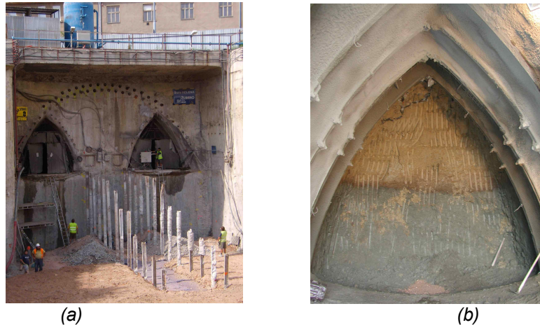
Fig.1 Exploratory adits situated in the tunnel top heading (a), left drift excavation with boundary of altered and non-altered Brno clay (b)
