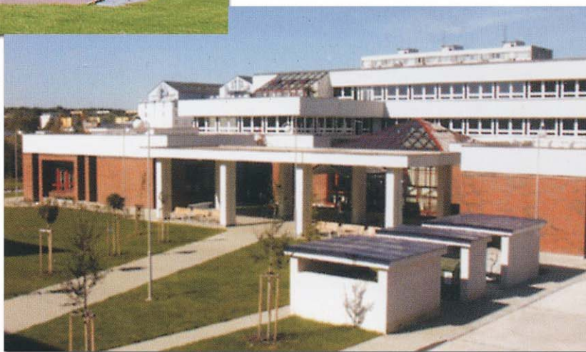
Building "B" (conference site)
